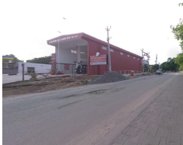
Figure 2. High-definition photo taken by the laser scanner showing the pavement with potholes
