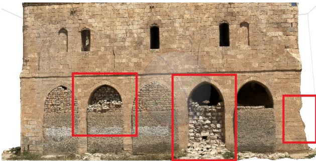
Figure 5. The deformed parts of the historical church
