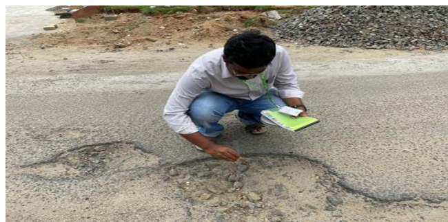
Figure 1. Pothole in the study stretch
